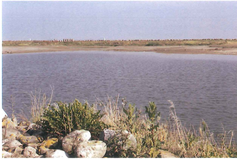
Figur 2. Nordøstlige del af lagunen. Den nye mole skimtes i baggrunden. Northeastern part of the lagoon. The new mole is seen in the background.
